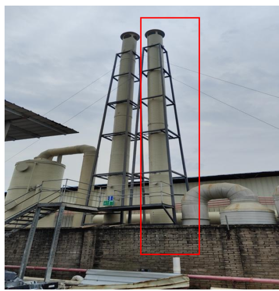
铜电解精炼线废气排放口DA010
